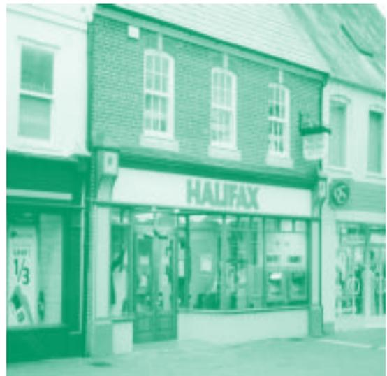
The top of the fascia should normally be well below the cills of the windows on the first storey. Fascia boards should be designed as an integral part of the shopfront avoiding reflective, garish or fluorescent colours and materials.
